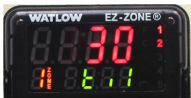
Fig. 5- The Watlow controller displays the time integral parameter.
